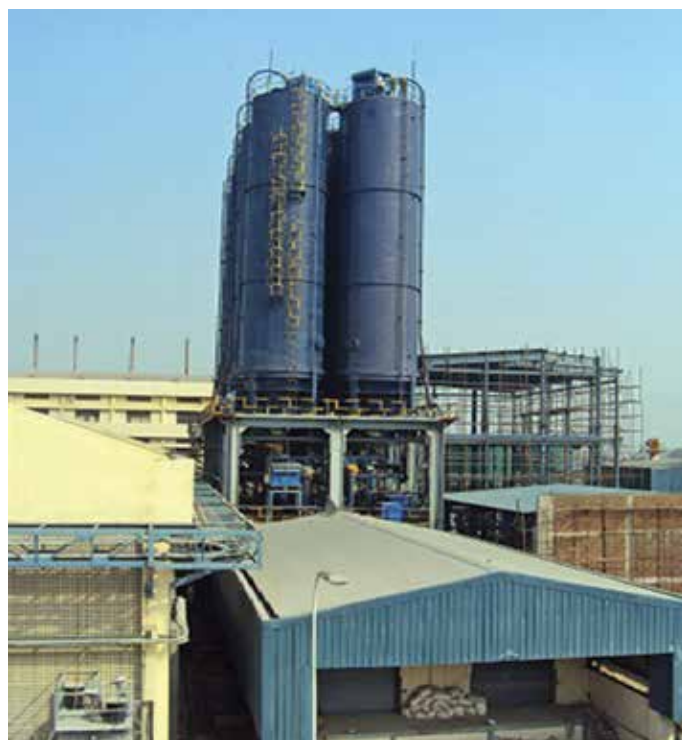
Silo System at Jainpur
