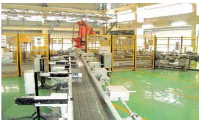
Automatic Filling line at Jainpur
